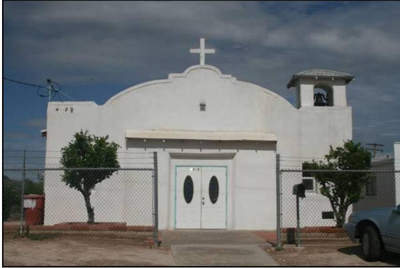
Mission San Lima, 2015 N. Calle Central, constructed 1930. (Photo by Clinco)
