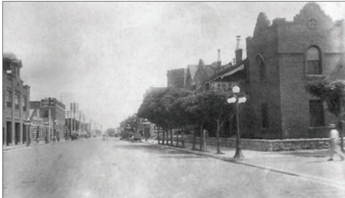
Sixth Avenue with the Willard Hotel, early 1900s. The Willard, later renamed the Pueblo Hotel (shown in the sketch above), was recently rehabilitated for offices and is a good example of adaptive reuse.
